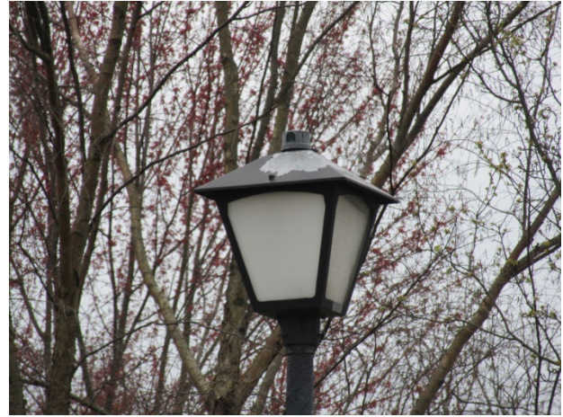
Finish deterioration at Chatsworth Court
