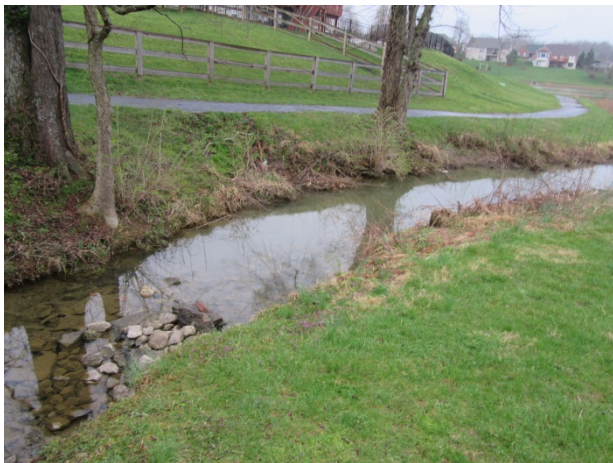
Central pond northern inlet channel overview
