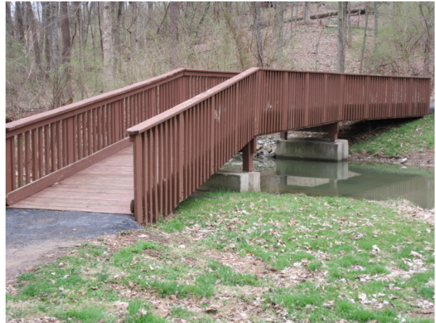
Eastern bridge overview
