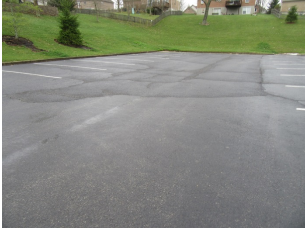
Pavement cracks
