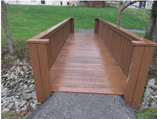
Northern bridge overview
