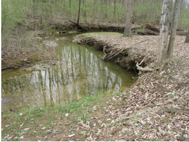
Erosion at central pond eastern inlet channel
