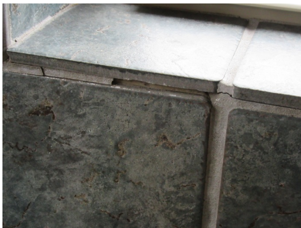
Grout deterioration
