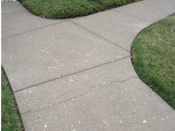
Sidewalk cracks
