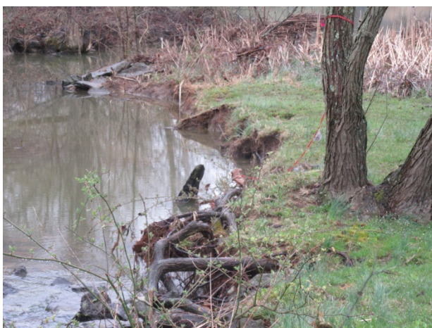
Western pond northeastern inlet channel erosion
