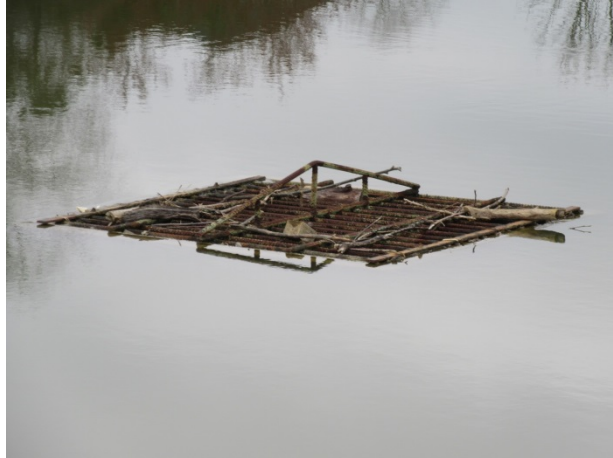
Central pond control structure overview
