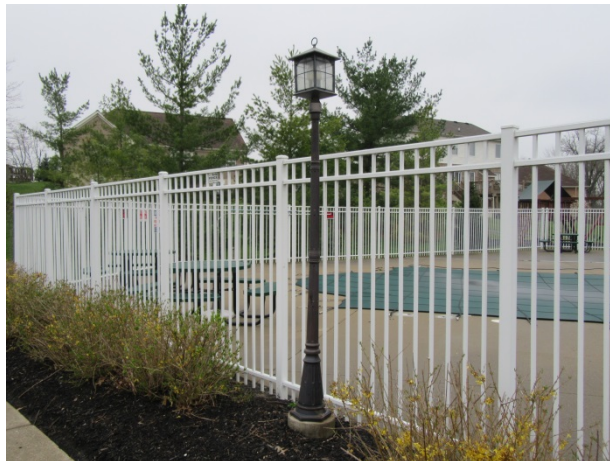
Light pole and fixture overview
