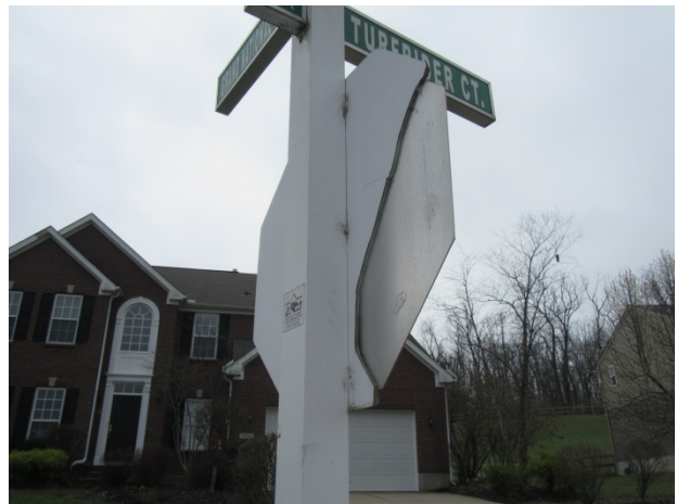
Damage at Turfrider Court
