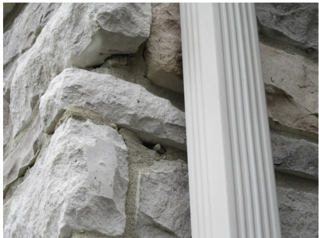
Mortar deterioration
