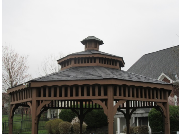
Roof and cupola overview
