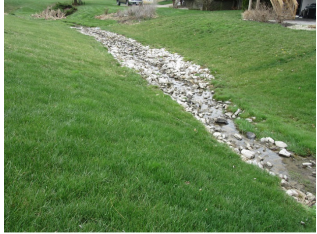
Overview of rip rap between Foxhunt and Wexford Drive
