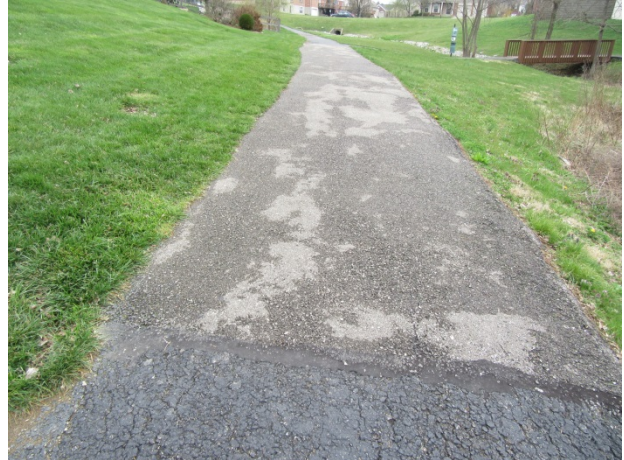
Partial replacement near northern bridge
