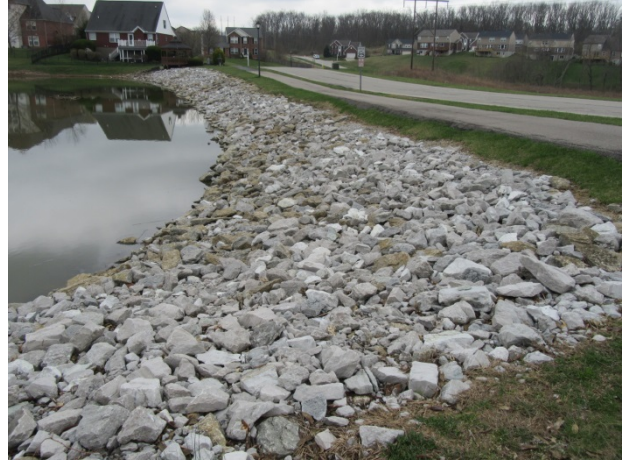
Overview of central pond southwestern shoreline rip rap
