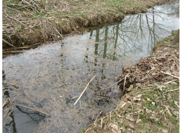
Organic accumulation at western pond southeastern inlet channel
