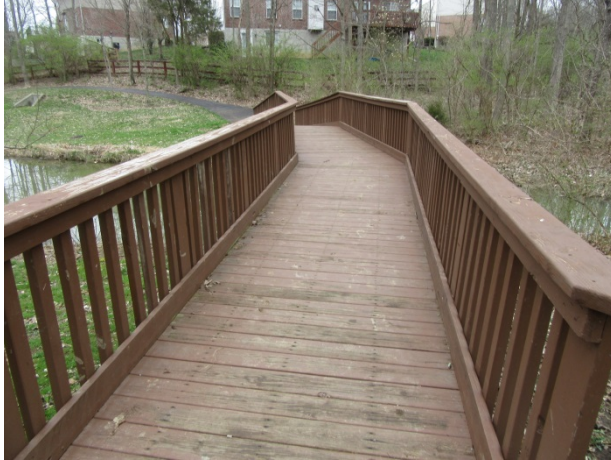
Eastern bridge walkway overview
