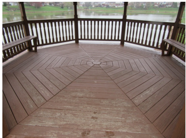
Deck board overview
