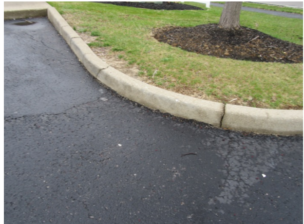
Curb cracks
